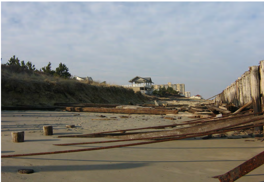
Photo 14. Coastal Bluff Community: View northward across eroded beach and damaged bulkhead in the South Beach Protected Zone to bluff with exposed sediments of the Manasquan Formation. (02-17-11)
